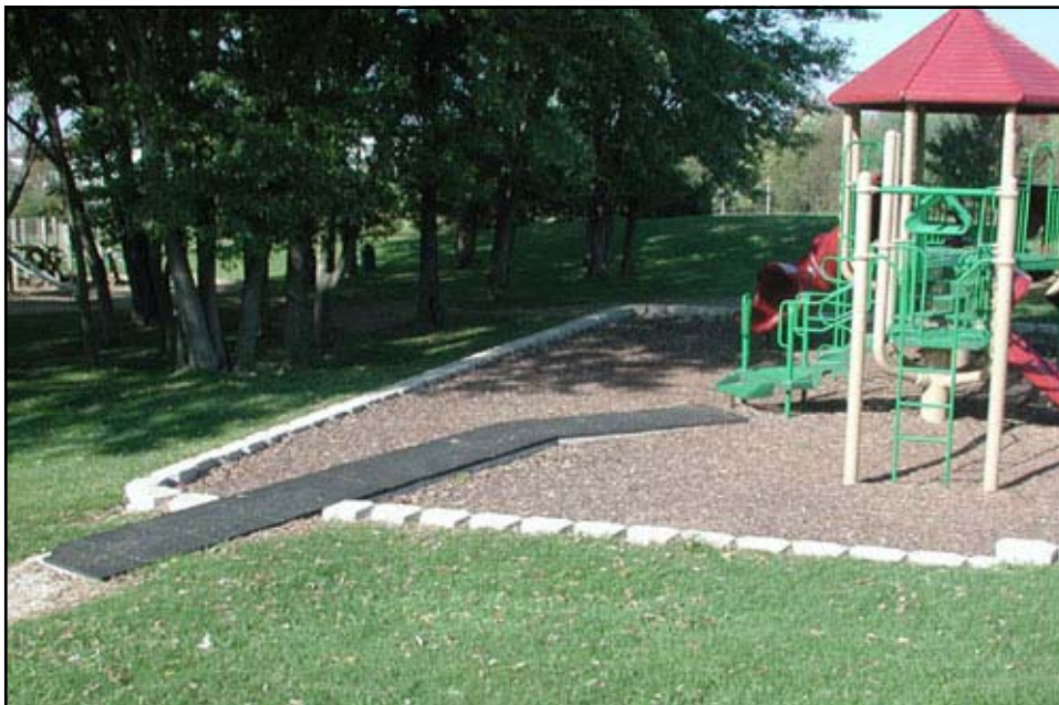
A rubber tile path affixed to a concrete base leads to a composite play structure.
