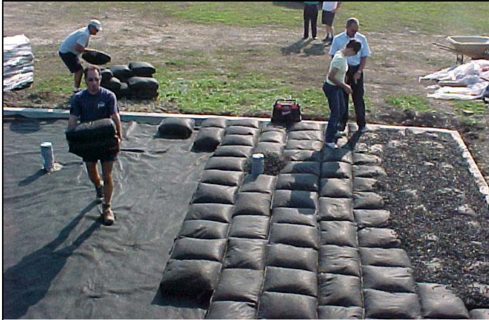
Two workers lay out bags filled with shredded rubber in a grid as part of the base for the SMART E Surfacing System. Two other workers fill the creases with loose rubber.
