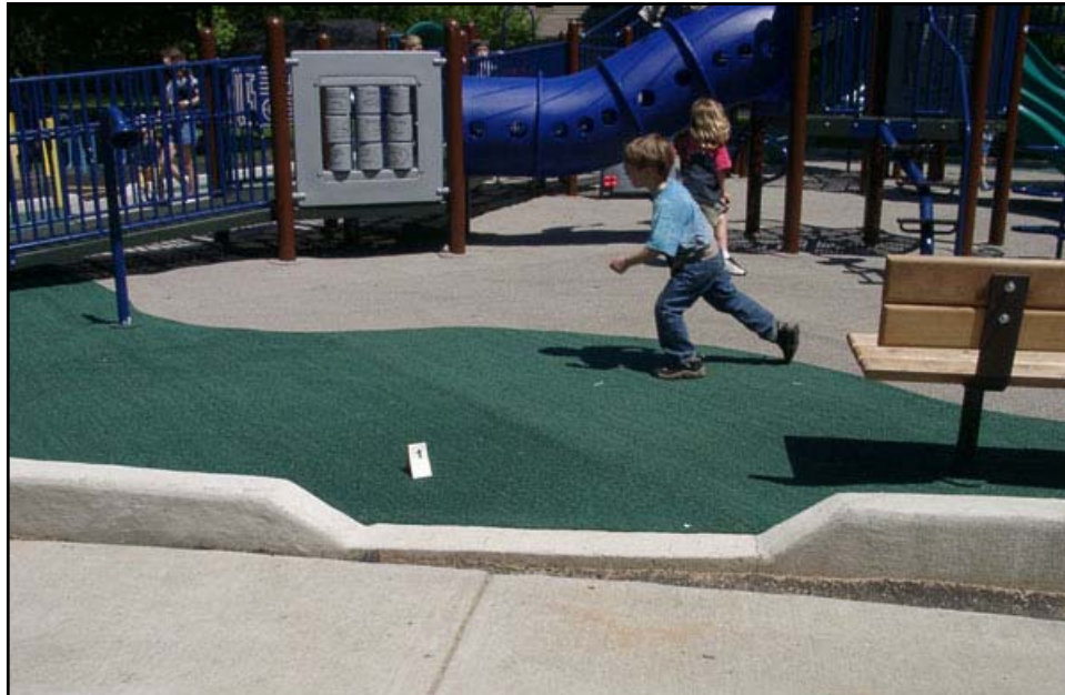
Curb cut from concrete sidewalk into unitary playground surface.
