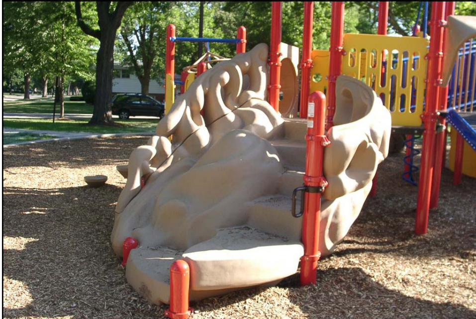
Transfer system to elevated composite play structure. Transfer system is molded plastic to look as if the child is climbing up a mountain trail.
