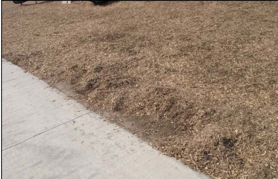
Concrete sidewalk treated with beveled edge into playground surface. Engineered wood fiber is filled to top of beveled edge. Some EWF has been kicked back to reveal beveled edge.
