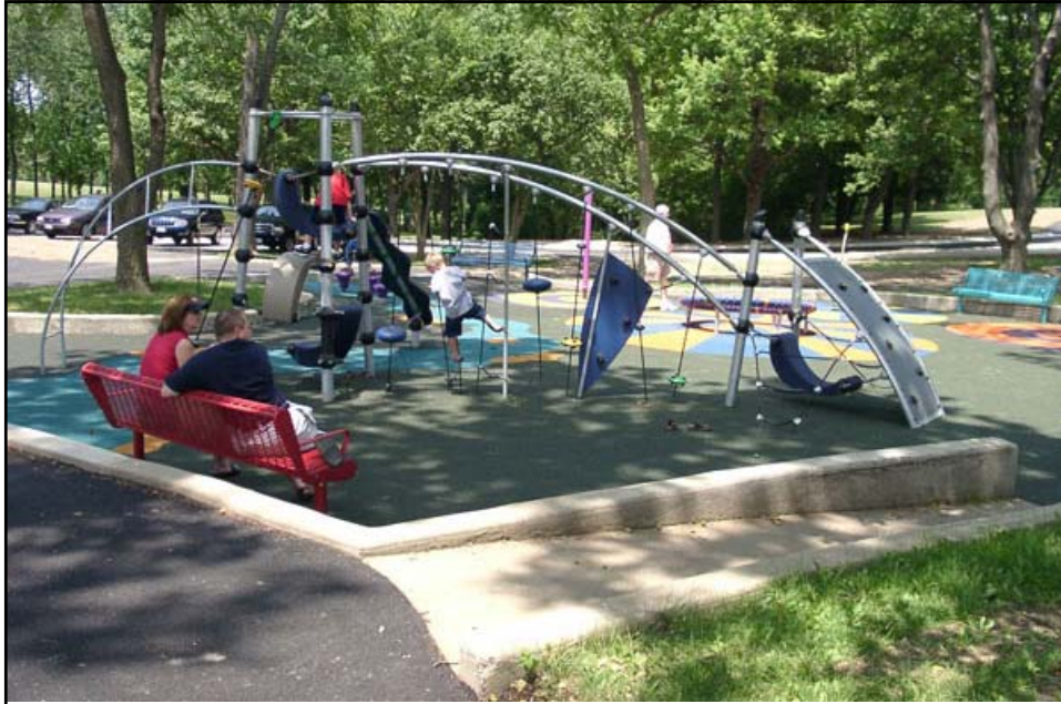
An asphalt route and landscape berm leads to a concrete ramp descending into a play area with unitary surfacing.
