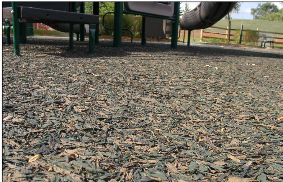
Large pieced shredded rubber is mixed with a binding product to make a unitary surface.
