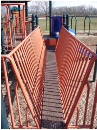
Right: An elevated platform wide enough for wheelchair passage connects the same two platforms of the elevated composite structure.
