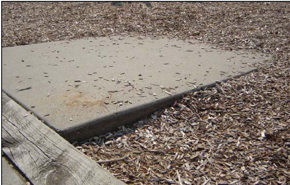
Concrete ramp extending into loose fill playground surface.
