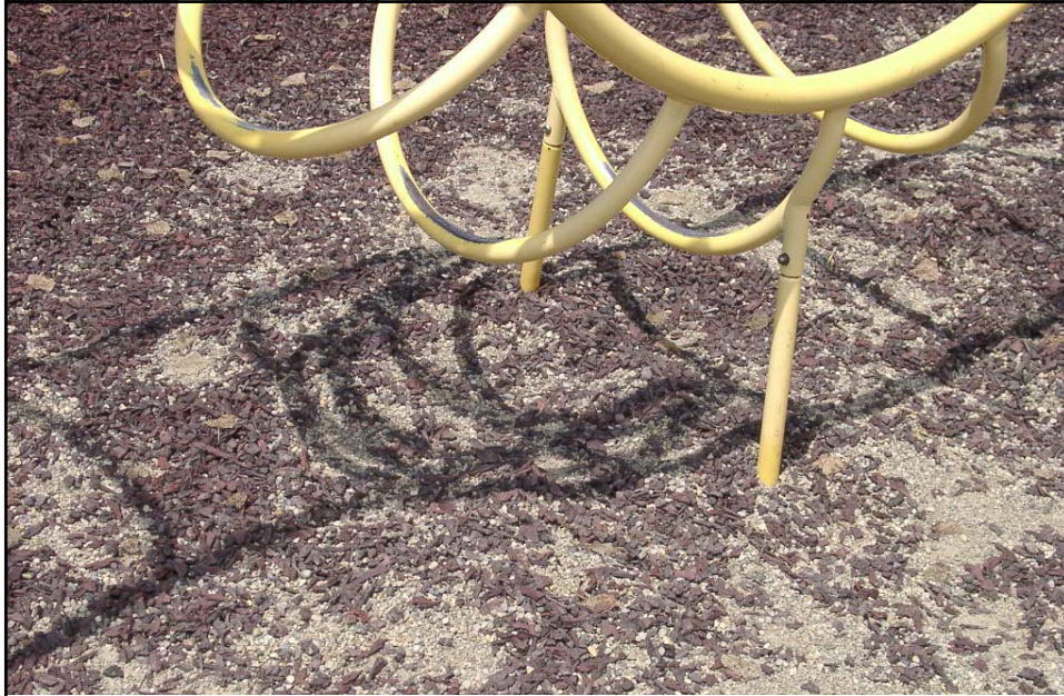
The gravel sub-base has mixed in with the shredded rubber playground surface under a climber.
