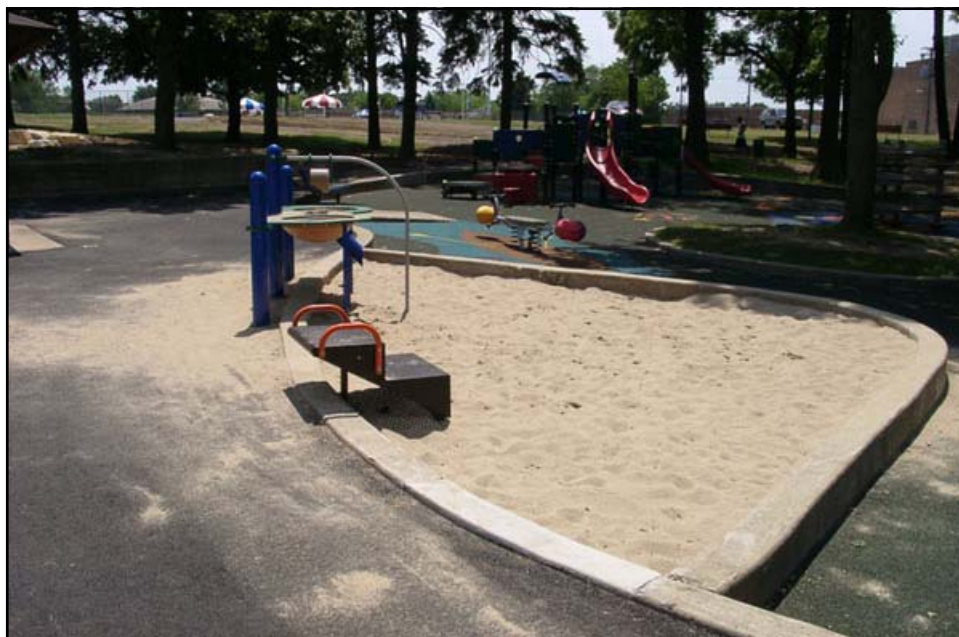
Sand area contained by concrete curb border. Sand table and transfer system adjacent.
