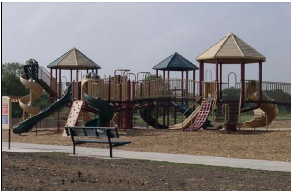
Large playground structure with engineered wood fiber surfacing and concrete sidewalk perimeter.
